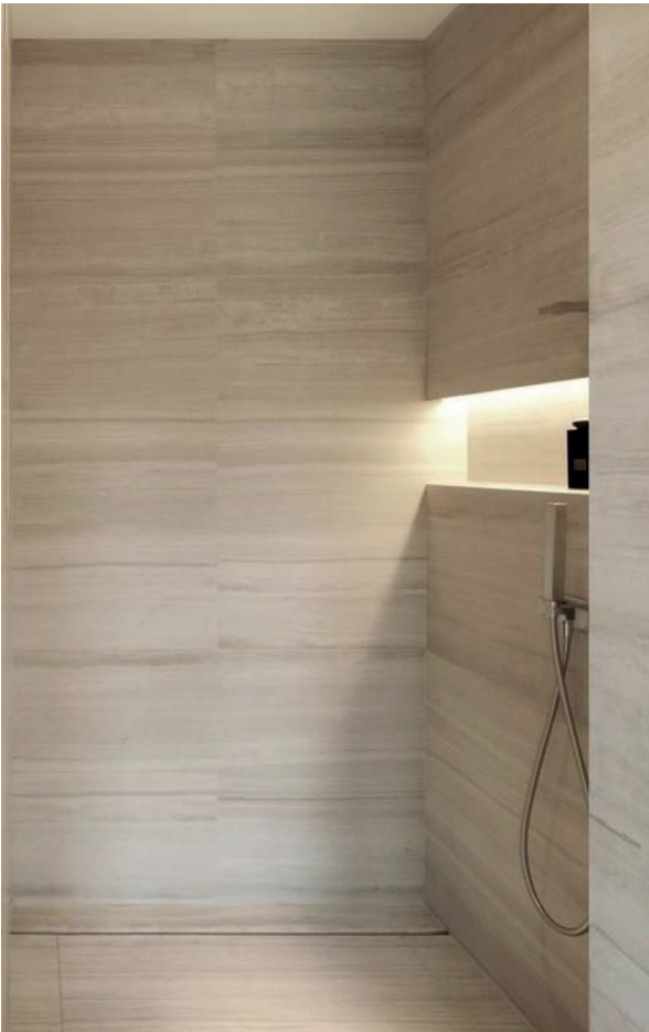
Built-in niche in showers with integrated LED lighting
